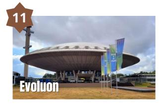
The Evoluon is a discus-shaped building, designed by the architects Louis Kalff and Leo de Bever. The futuristic flying saucer-like dome measures 77 m in diameter and the concrete of the dome is held in place by 169 kilometers of tension cable. The building is used for exhibitions and as a conference and event centre. It was designated as a national monument in 2018.
